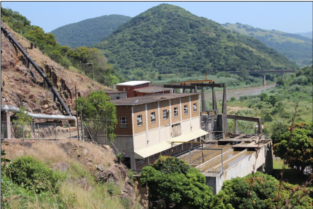
St Helens Rock pump station
