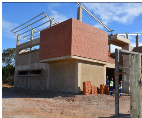
Construction in progress at the new Disaster Centre site
